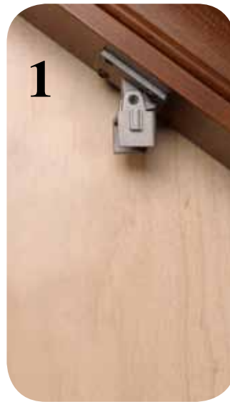
1 Install Clip To Handrail and Tread
