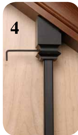
4 Slide Shoe In Place And Tighten
